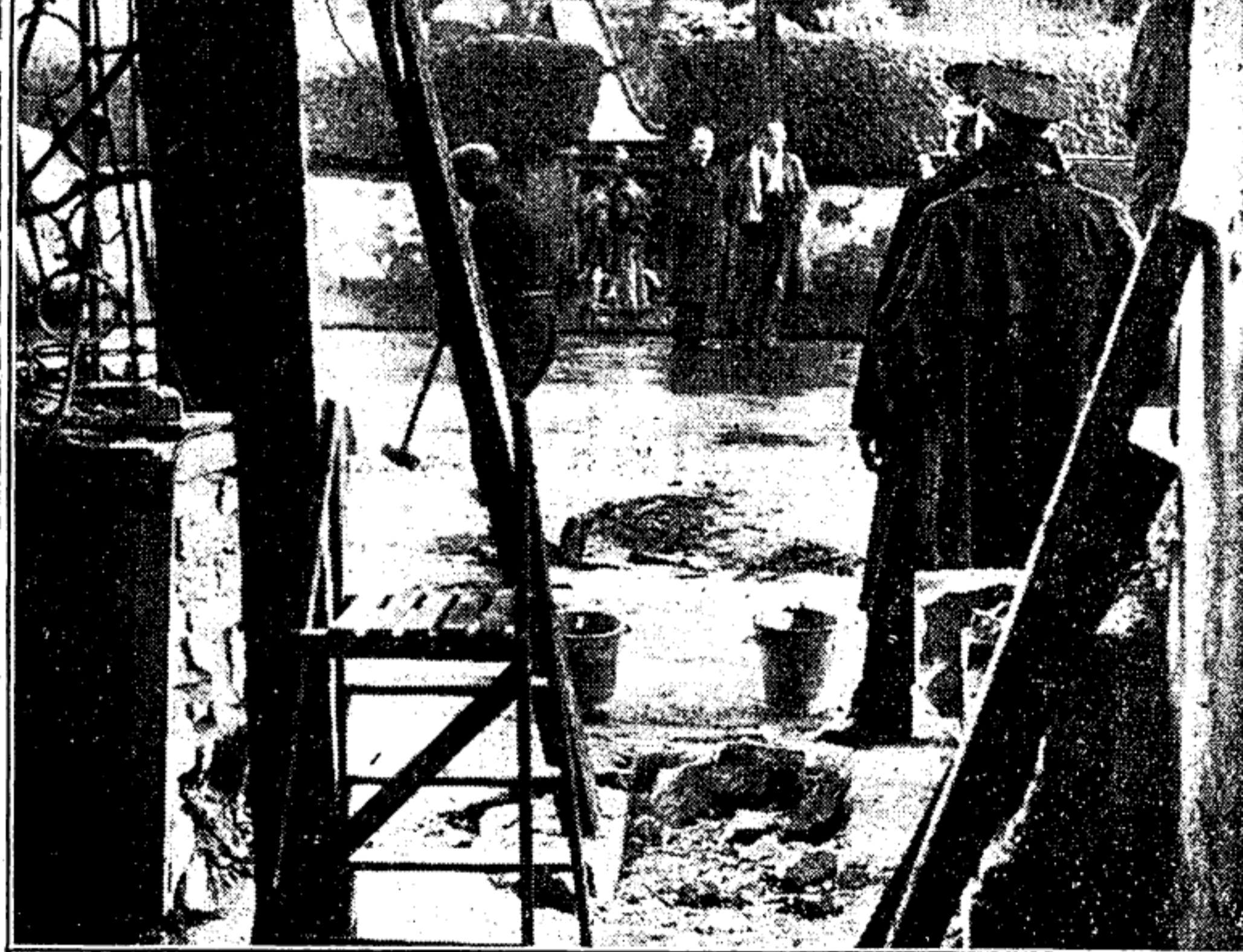
Our photographer took this picture looking out from the barrack hallway and showing the opening where the door, door frame and porch with four pillars had been. The sloping pathway on the far side leads to the house of Mr. O. Reynolds, which suffered much damage. Further up this hill is Moate Brae, where the raiders stationed themselves when they exchanged shots with the police.
